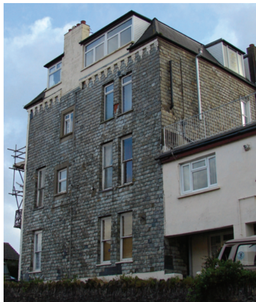
Slate hanging on the south west gable of Adelaide Terrace
