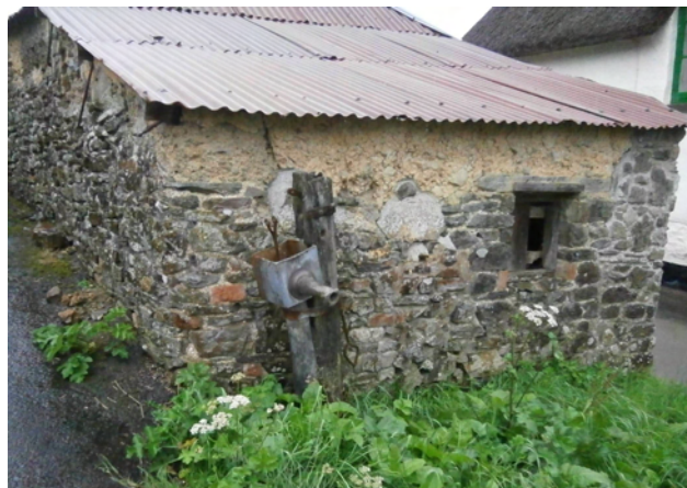
One of the two water pumps which survive in the village.
