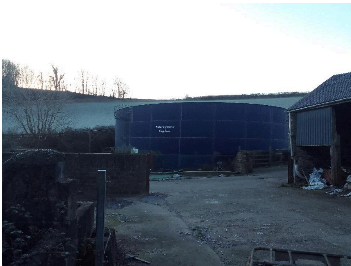
Figure 4.1 Slurry Tank (North Devon Council)
