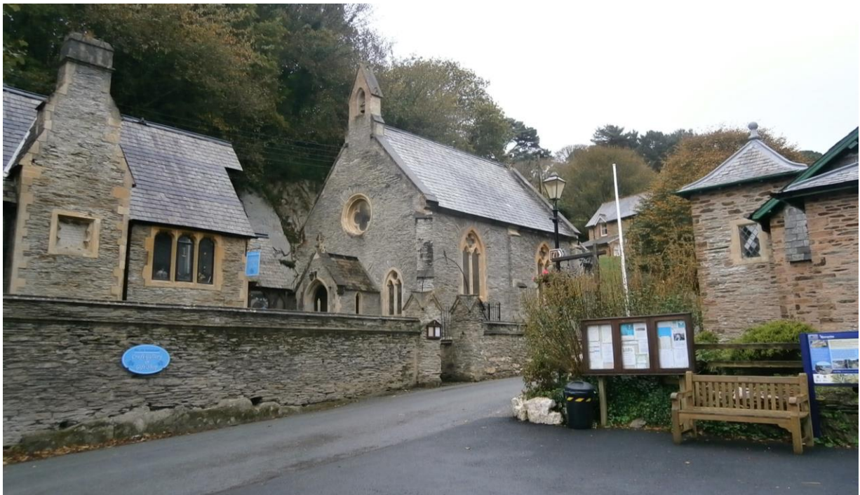
The Parish Church and art gallery in the former schoolroom to the left form a distinctive group, together with the Memorial Hall to the right.
