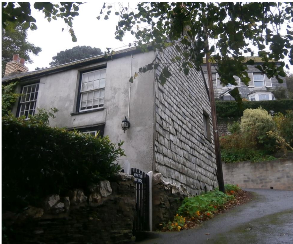
Looking uphill from Myrtle Cottage at slate hung walls and gables, and sash windows.
