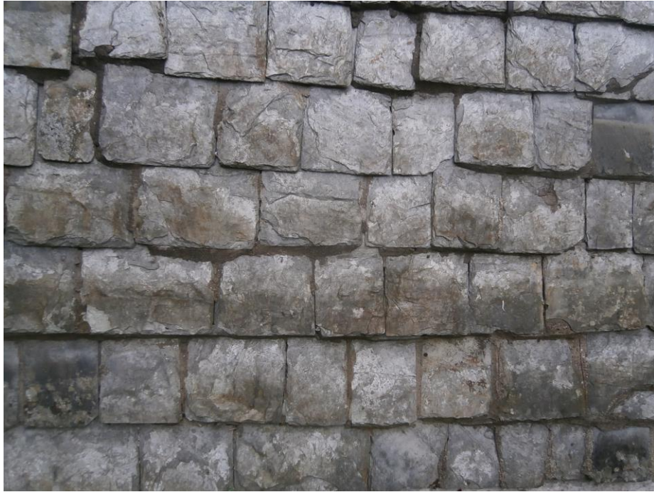
Slate hung walls are a distinctive and functional feature of the group of houses in the north-eastern part of the Conservation Area.
