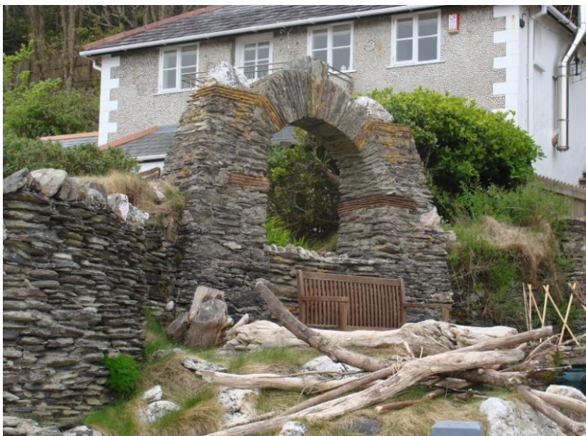
The garden walls at Smugglers Cottage are an extravagant example of local stone walling, incorporating clay tile bands for reinforcement and decorative use of white spar.
