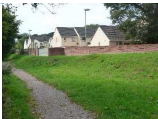
Figure 8-2: Flood wall on top of embankment
