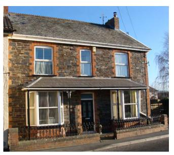
orange tinted bands. The material is reasonably durable but it does not work well. As a result the masonry which it forms is usually rendered as it was not thought to give a highly attractive result.
