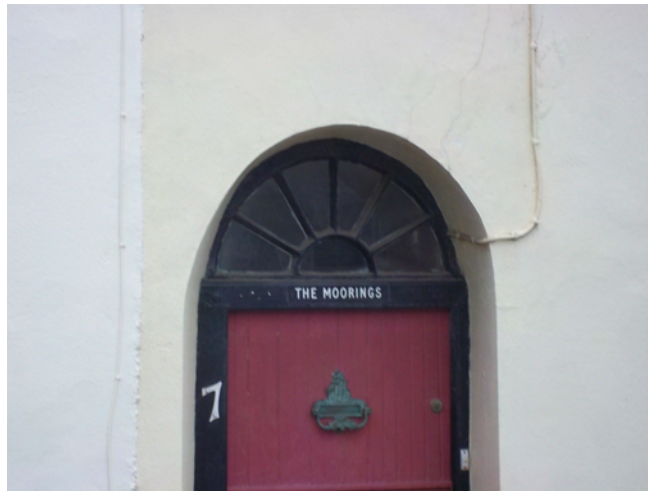
Example of a fanlight above the front door of a property at Lane End Road
