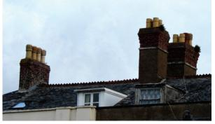
**4.3** Alterations damage the distinctive character of chimneys by the application of smooth, crisp render that hides stonework or flattens an uneven surface. Removal of drip slates and historic pots also detracts from the character of the area and should be avoided wherever possible.
